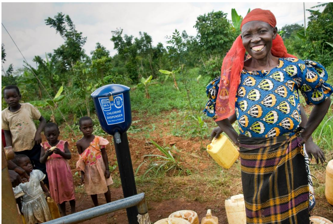
A woman and children are standing next to a chlorine dispenser installed at a water source in a village in Kenya.
