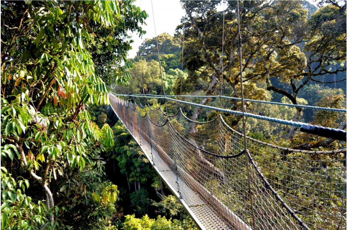
Footbridge suspended over a jungle in Rwanda.
