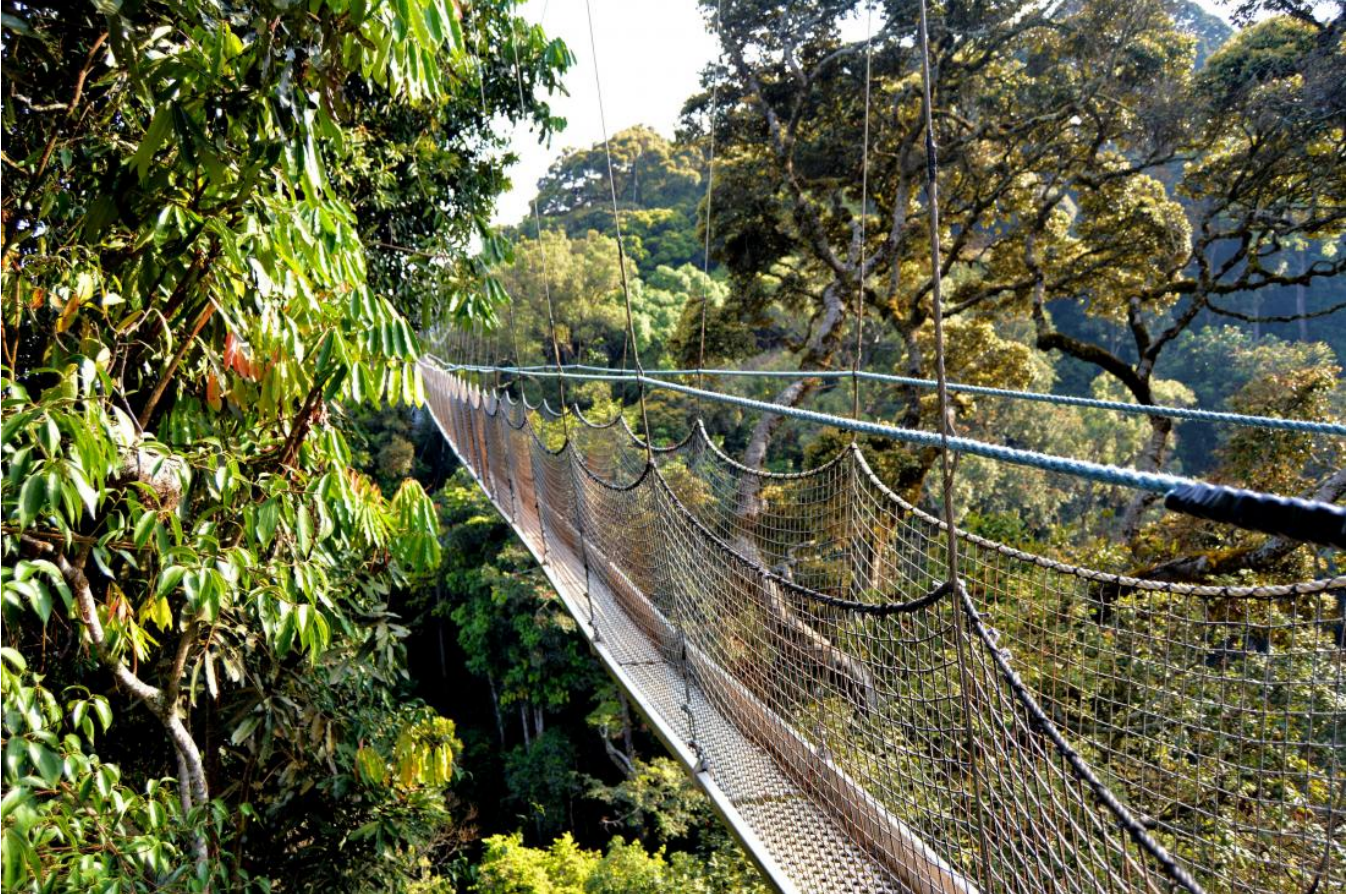
Footbridge suspended over a jungle in Rwanda.
