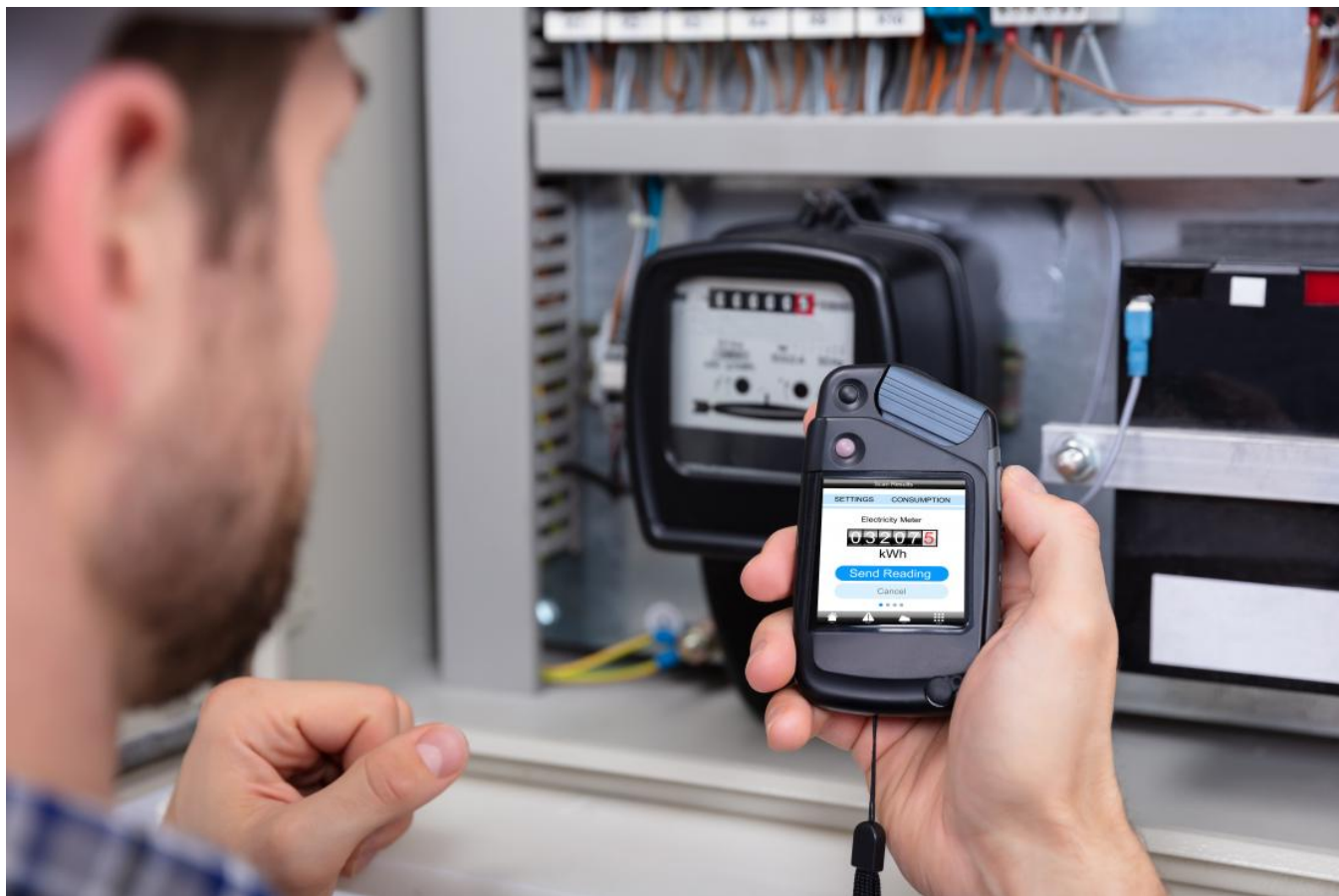
A technician reads a meter.
