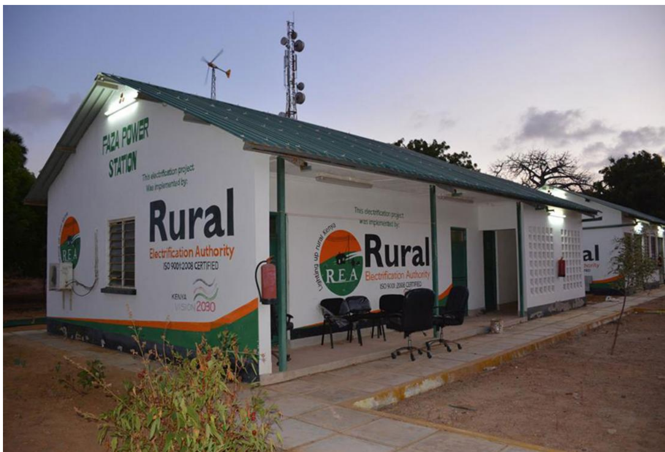
A power station managed by Kenya's Rural Electrification Authority
