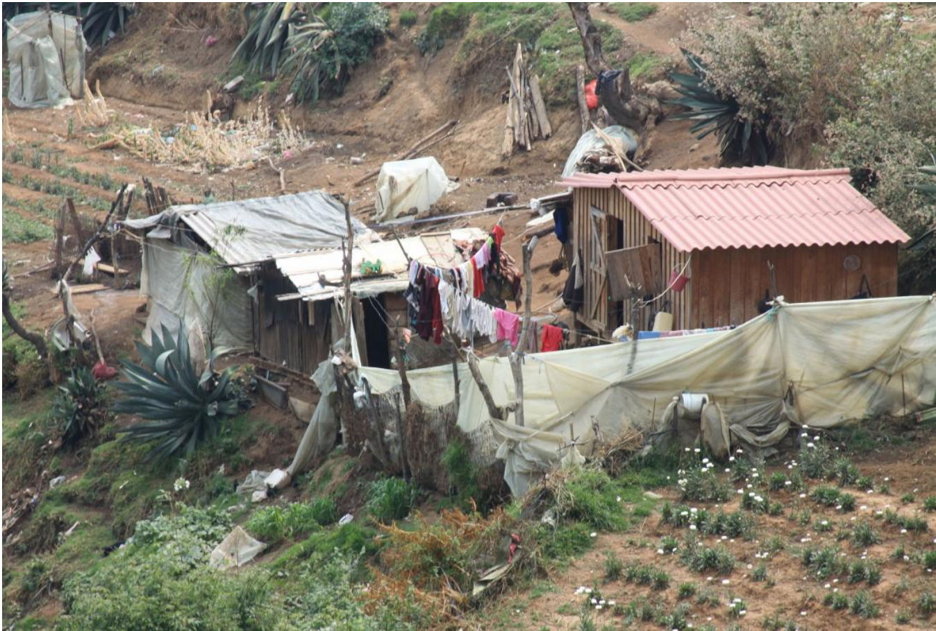
Slum housing in Mexico
