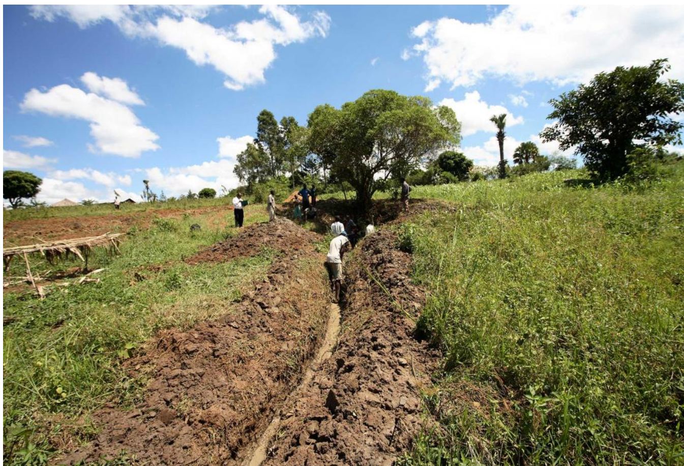
Introducing irrigation to central Kenya
