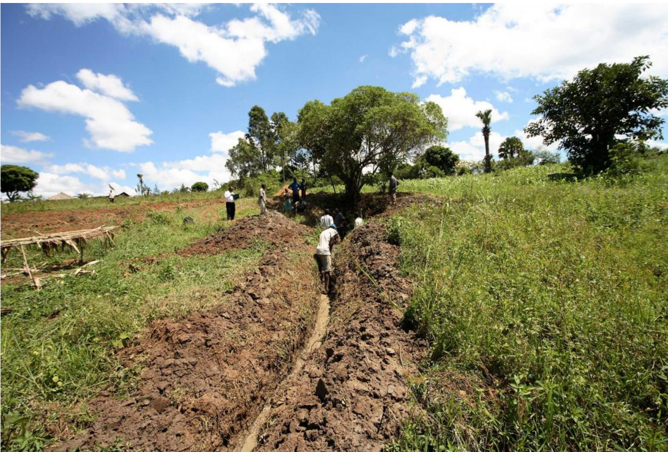
Introducing irrigation to central Kenya
