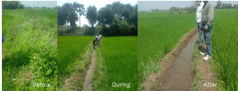
Figure A1: Images Before, During, and After Channel Construction
